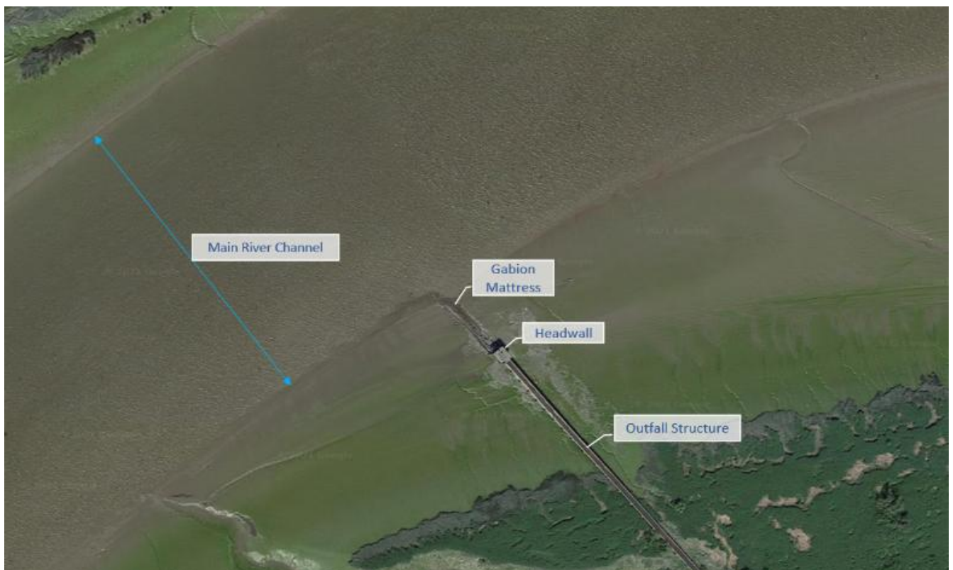
FIGURE 3-13: OVERVIEW OF OUTFALL STRUCTURE
